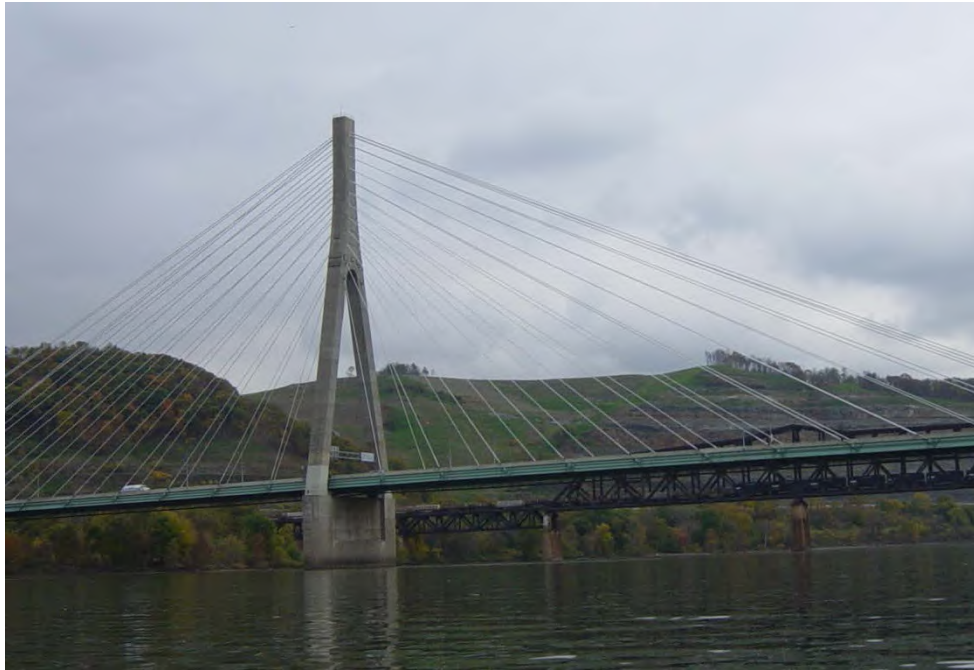
Figure 3.1.20 Cable-Supported Bridge: Cable Stayed
