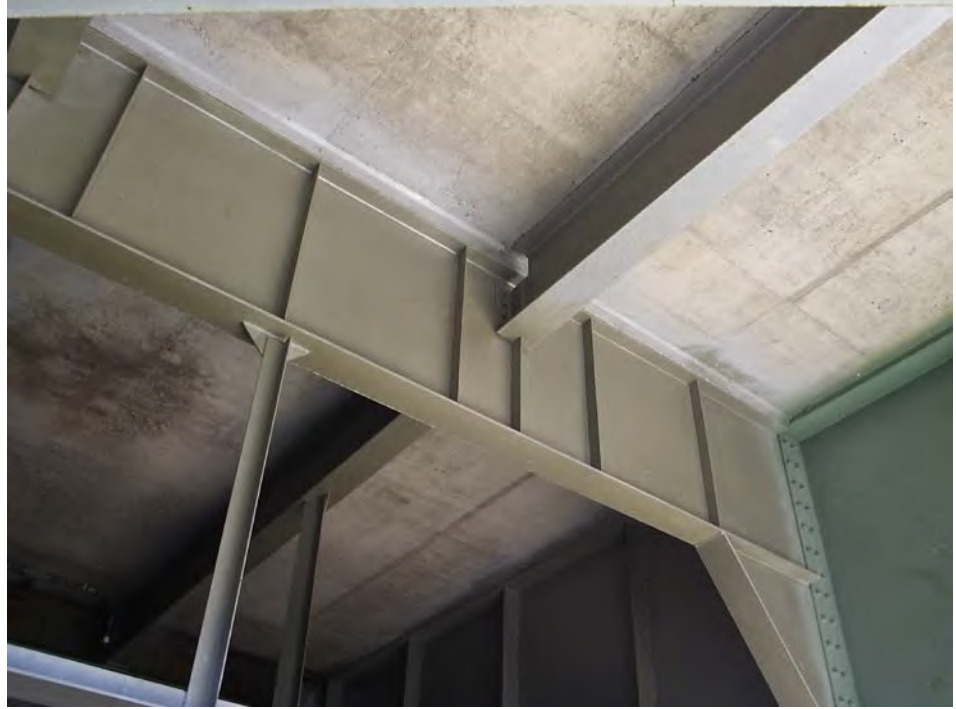
Figure 3.1.29 Underside View of a Bridge Deck
