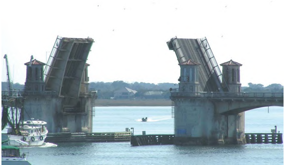
Figure 3.1.59 Bascule Bridge
