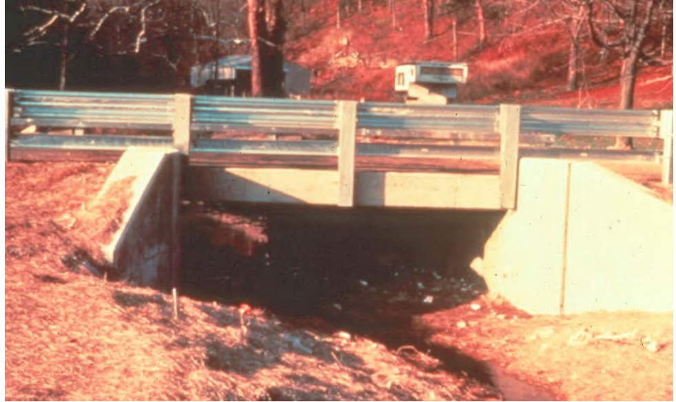
Figure 3.1.44 Slab Bridge
