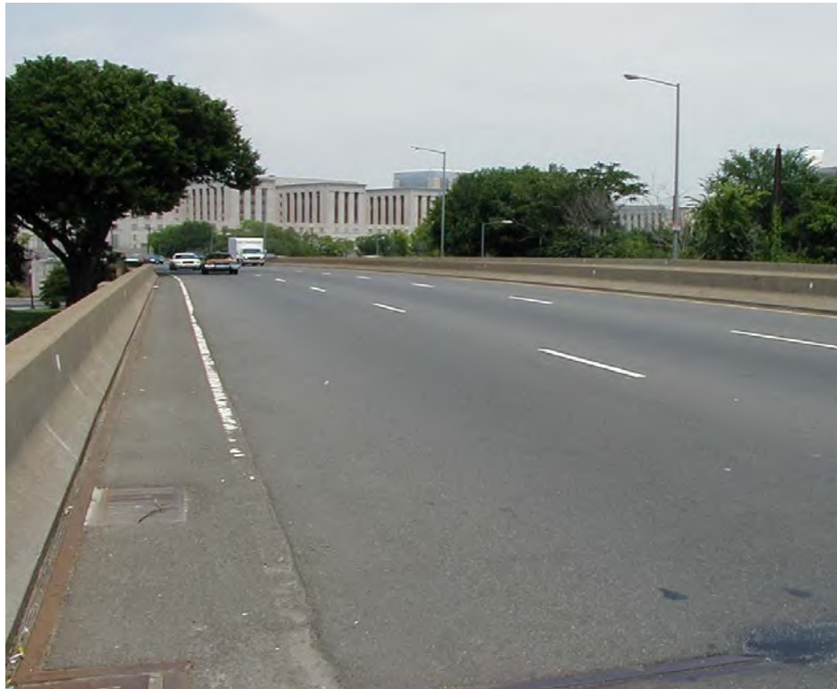
Figure 3.1.36 Asphalt Wearing Surface on a Concrete Deck
