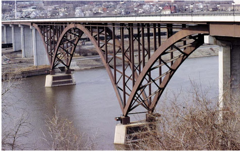
Figure 3.1.64 Main Supporting Members of Deck Arch
