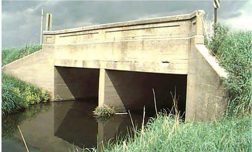
Figure 3.1.83 Rigid Culvert
