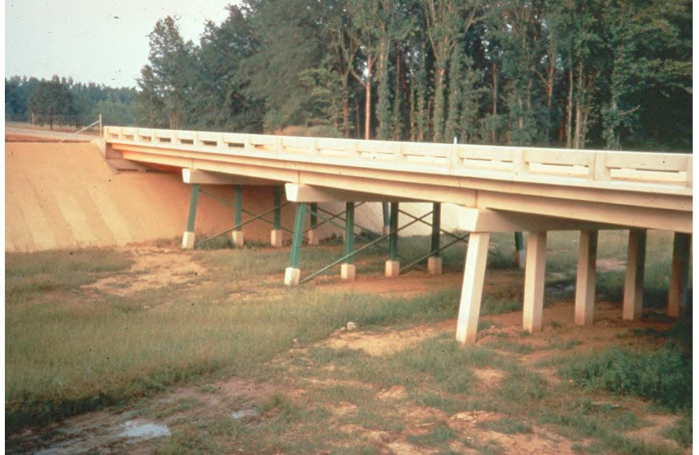
Figure 3.1.81 Pile Bent
