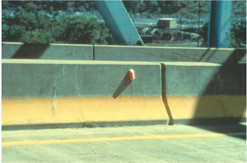
Figure 3.1.40 New Jersey Barrier
