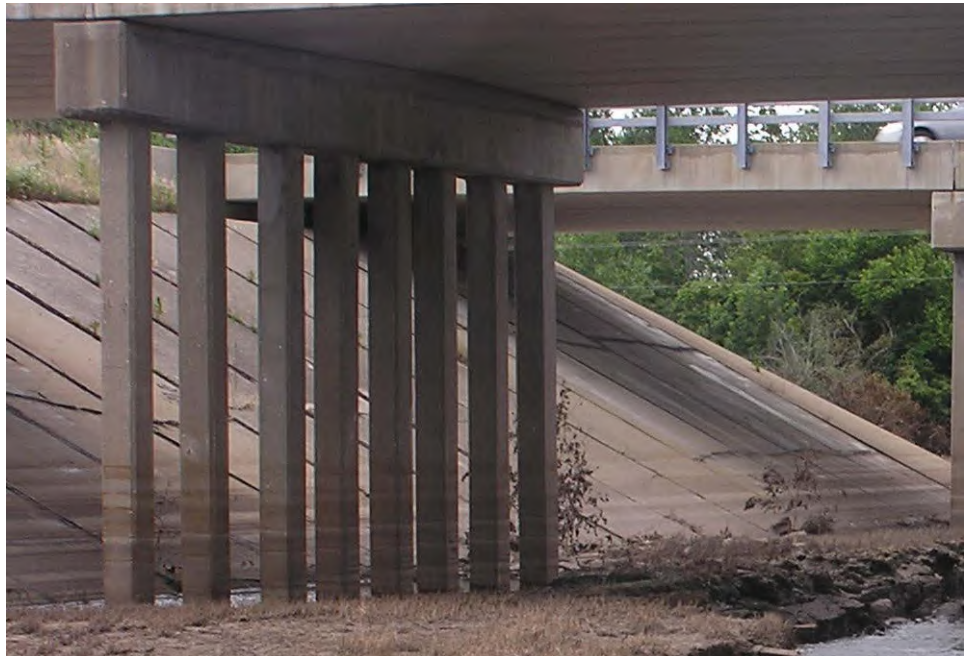
Figure 3.1.10 Concrete Pile Bent
