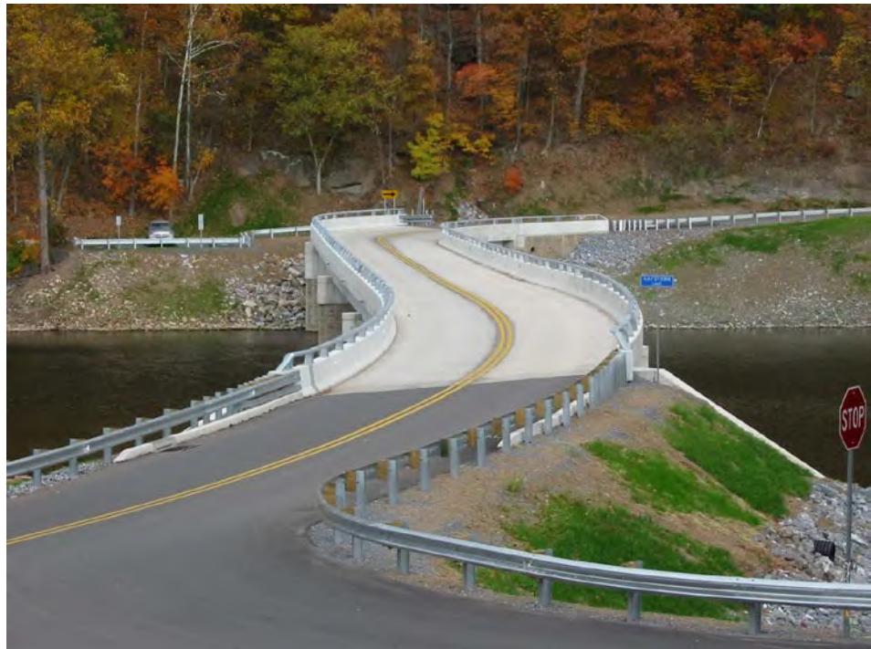
Figure 3.1.28 Bridge Deck with a Smooth Riding Surface
