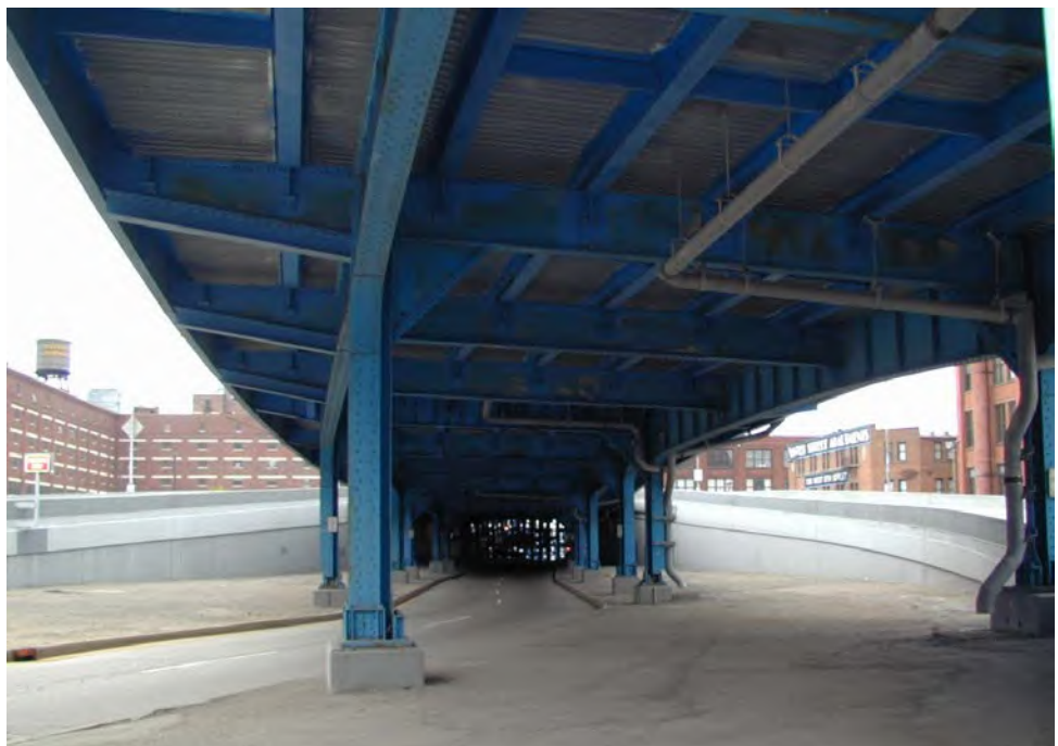
Figure 3.1.80 Column Bent
