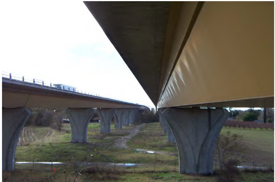
Figure 3.1.51 Box Girder Bridge
