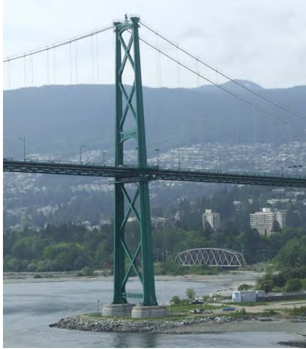
Figure 3.1.57 Suspension Bridge
