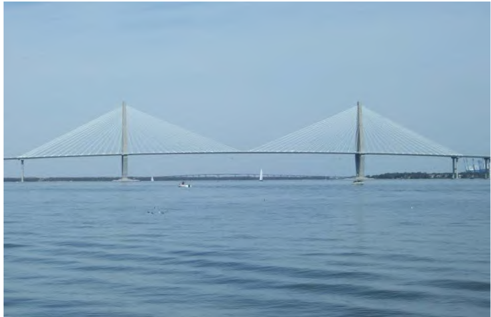
Figure 3.1.58 Cable-stayed Bridge
