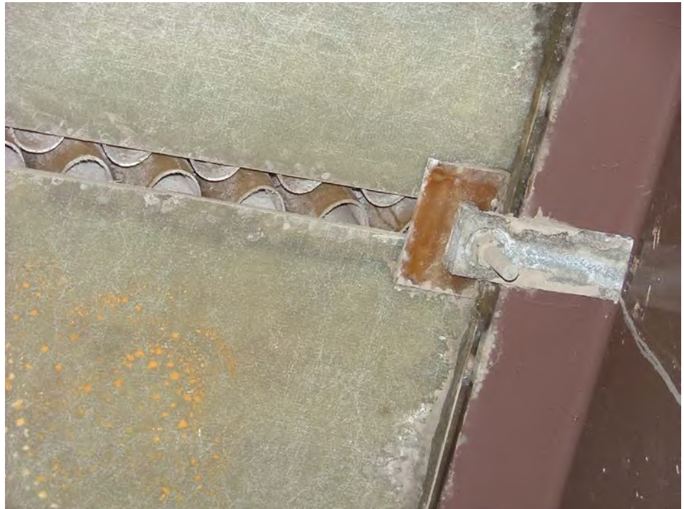
Figure 3.1.35 Fiber Reinforced Polymer (FRP) Deck
