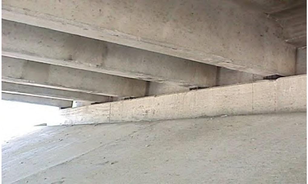
Figure 3.1.72 Stub Abutment
