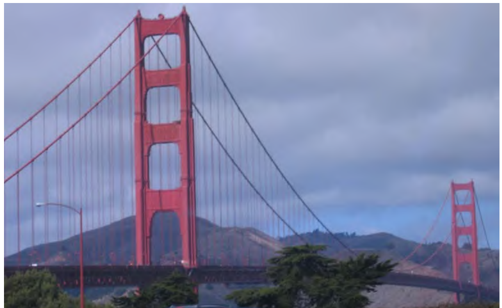
Figure 3.1.19 Cable-Supported Bridge: Suspension Cables and Hangers
