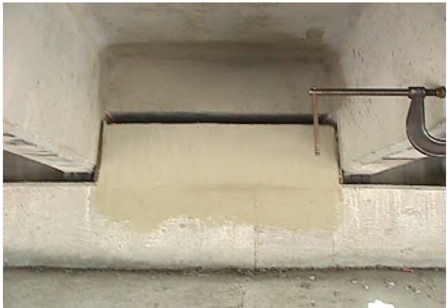
Figure 3.1.49 Tee Beam Bridge
