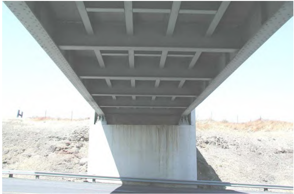
Figure 3.1.47 Girder Floorbeam Stringer Bridge
