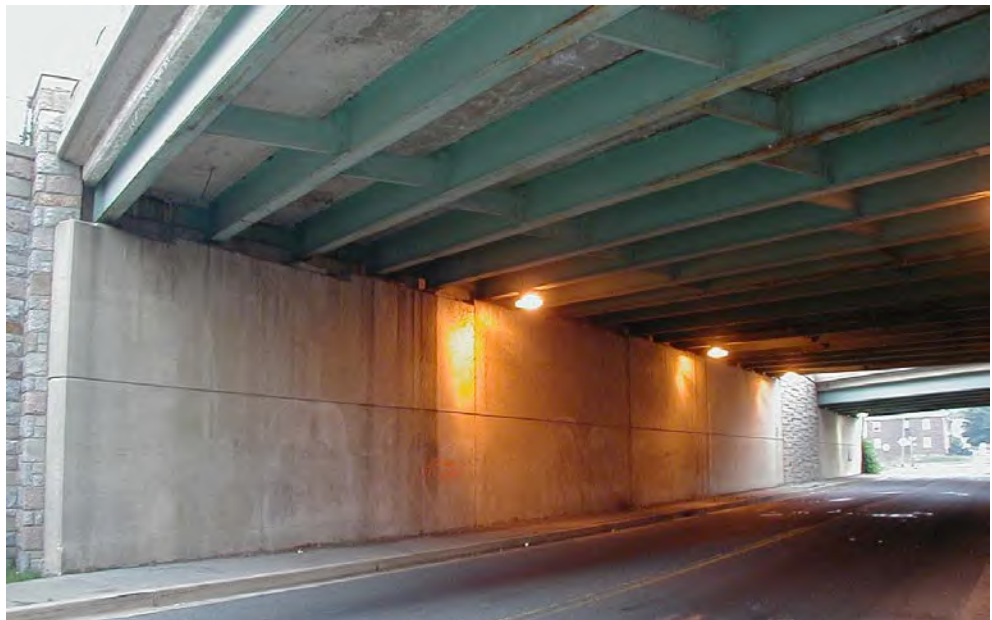
Figure 3.1.71 Cantilever Abutment (or Full Height Abutment)
