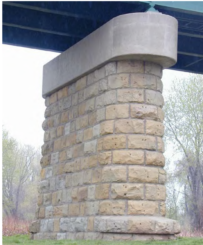
Figure 3.1.76 Solid Shaft Pier
