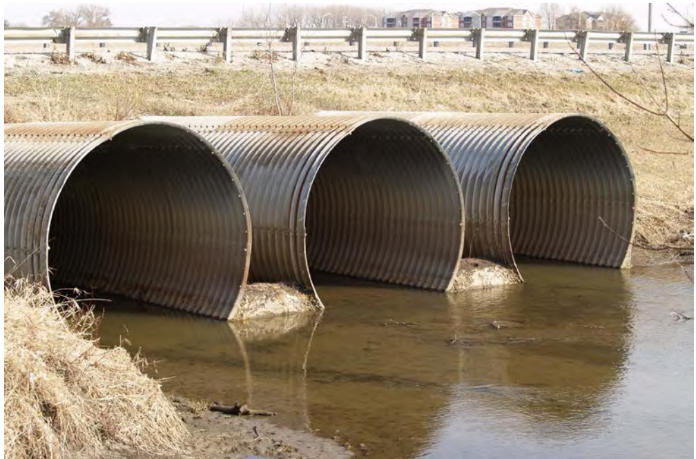
Figure 3.1.84 Flexible Culvert
