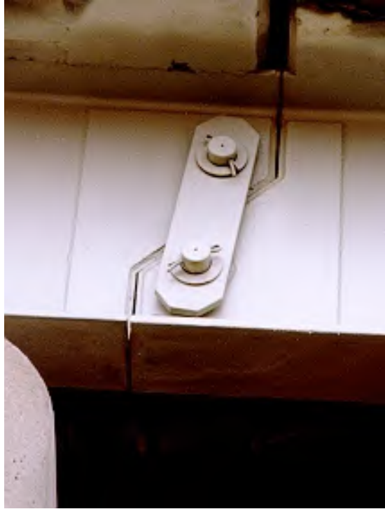
Figure 3.1.26 Pin and Hanger Assembly
