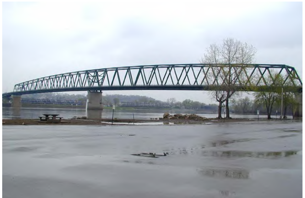
Figure 3.1.53 Through Truss Bridge
