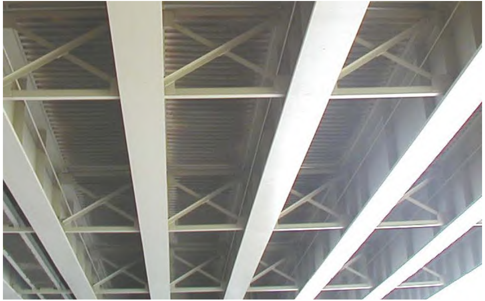
Figure 3.1.66 Cross or X-Bracing
