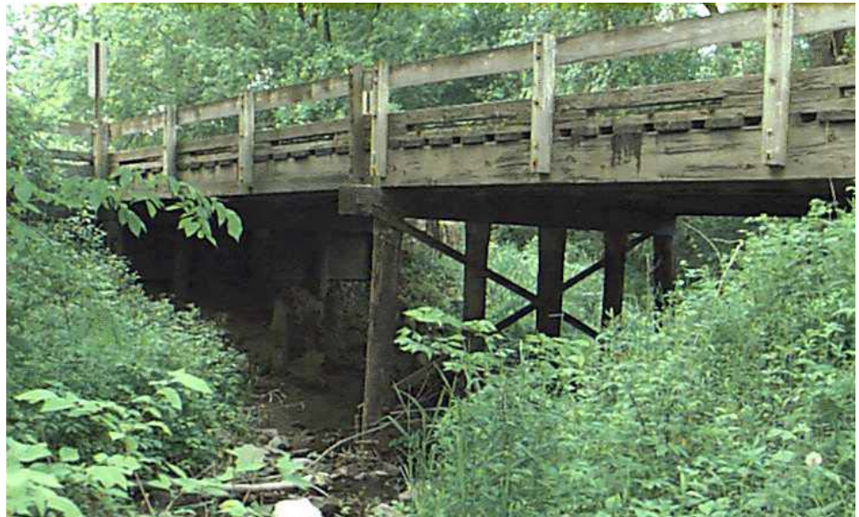
Figure 3.1.45 Beam Bridge
