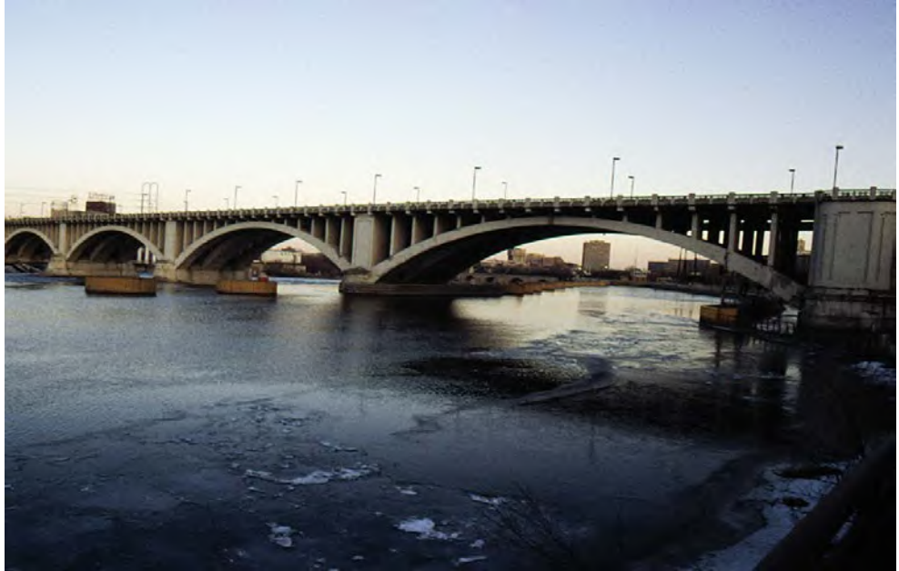
Figure 3.1.54 Deck Arch Bridge
