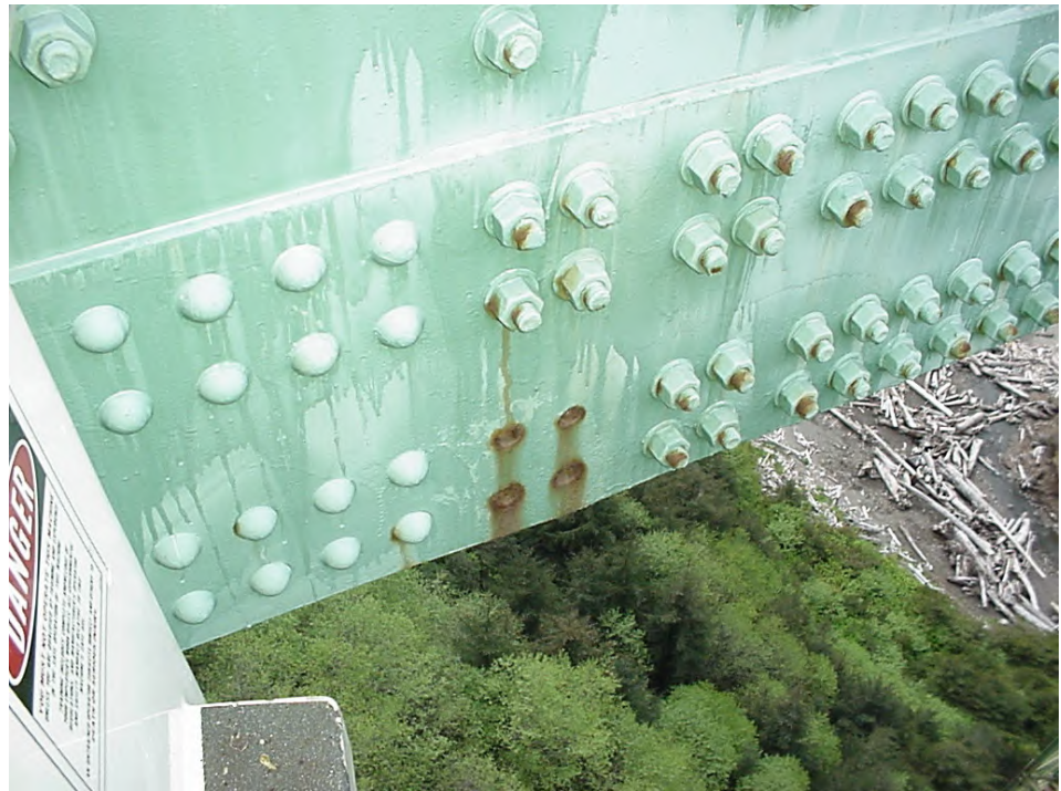
Figure 3.1.24 Shop Rivets and Field Bolts
