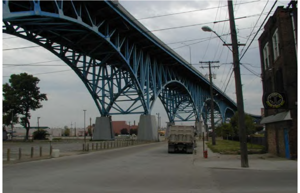
Figure 3.1.52 Deck Truss Bridge
