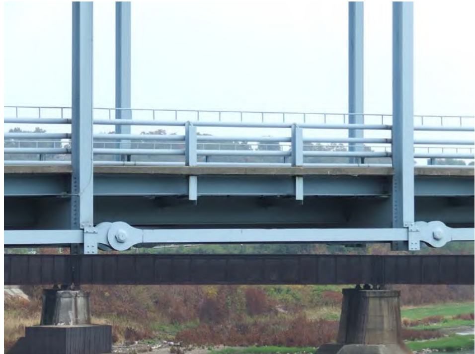
Figure 3.1.22 Pin-Connected Eyebars
