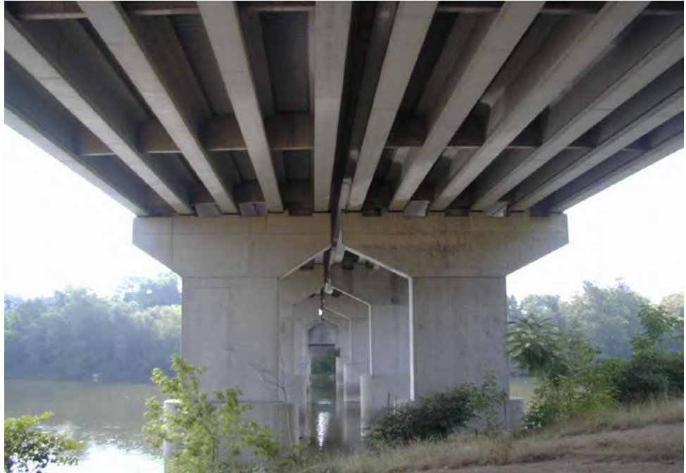
Figure 3.1.79 Cantilever or Hammerhead Pier
