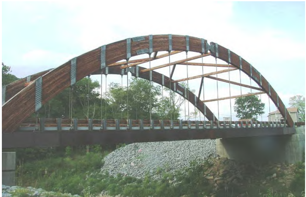
Figure 3.1.55 Through Arch Bridge
