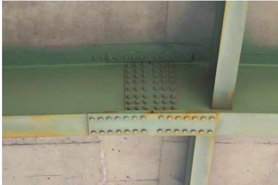
Figure 3.1.27 Bolted Field Splice
