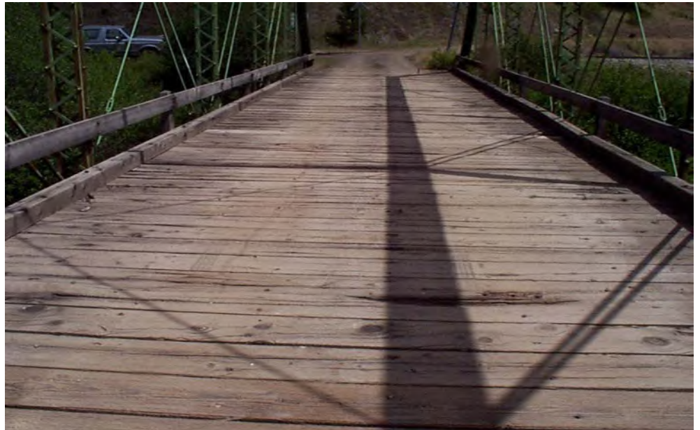
Figure 3.1.32 Plank Deck
