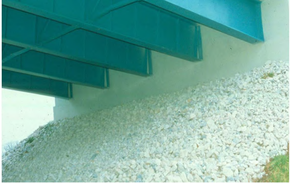
Figure 3.1.74 Integral Abutment
